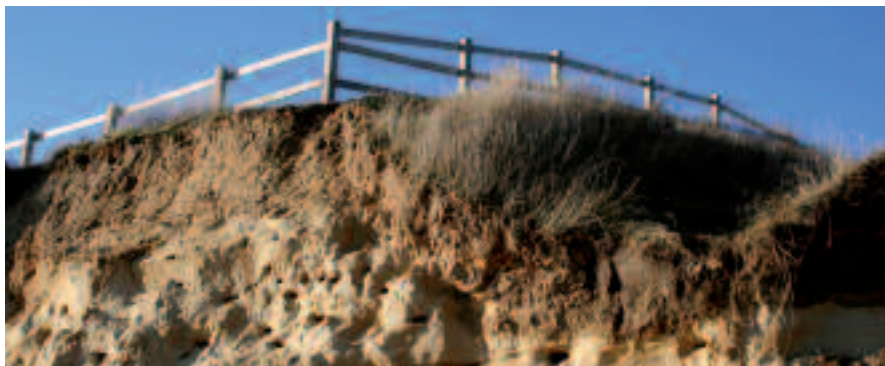
A fence on an eroded cliff top
